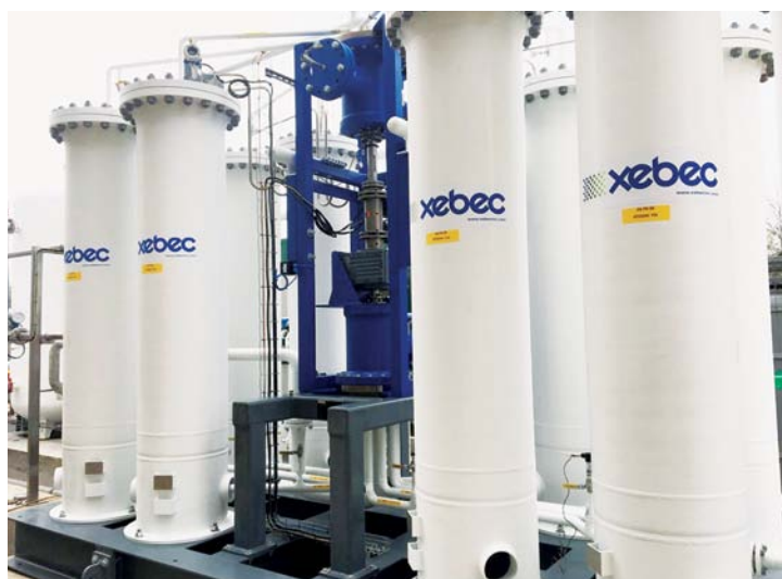
A Xebec PSA/pressure swing adsorption installation in France. Installation employing the company's new fast-cycle designs in Europe are already achieving the new performance levels, the company says.
